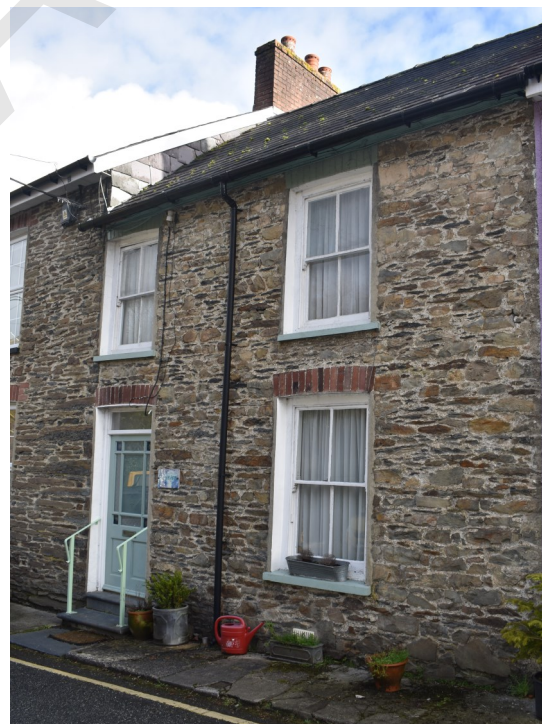
Fig. 2 Traditional cottage with original windows, slate roof, slate steps, traditional style replacement door
