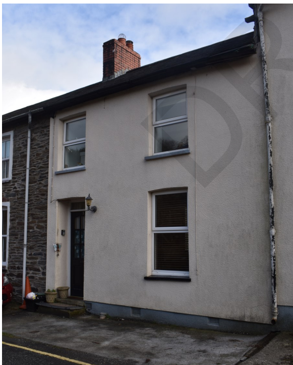
Fig 1 Traditional cottage with new windows, door, concrete render, fibre roof tiles, concrete steps
