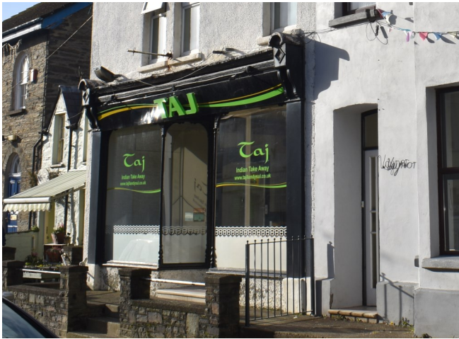
Fig. 12 An historic shopfront where the signage could be improved
