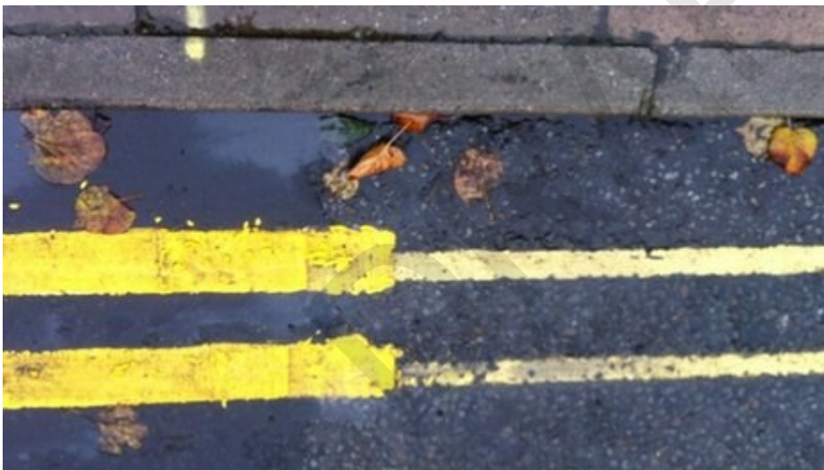
Fig. 27 Double yellow lines can be more subtle in conservation areas. (Louth, Lincs. Photo: BBC News)
