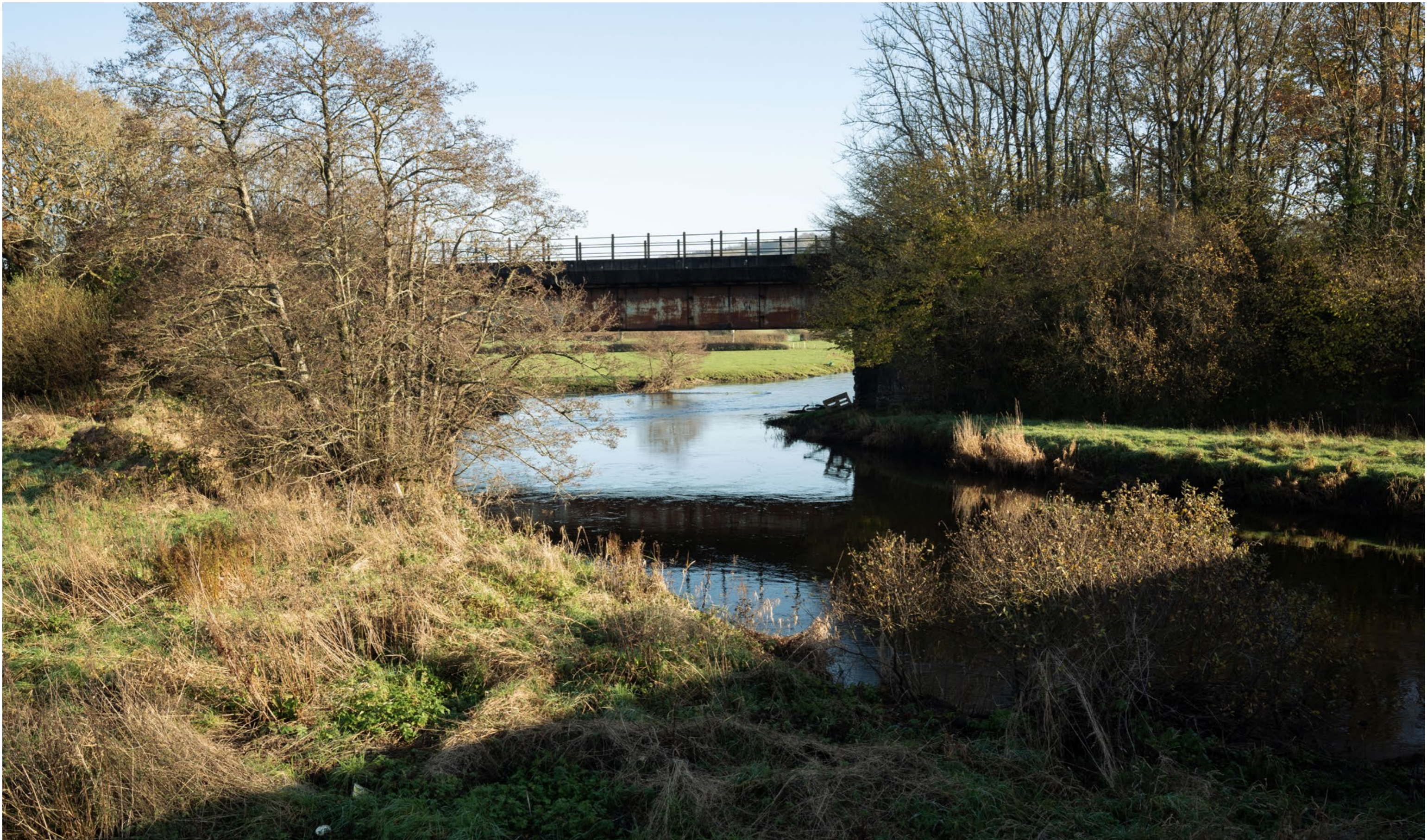
Dismantled railway bridge and River Teifi
