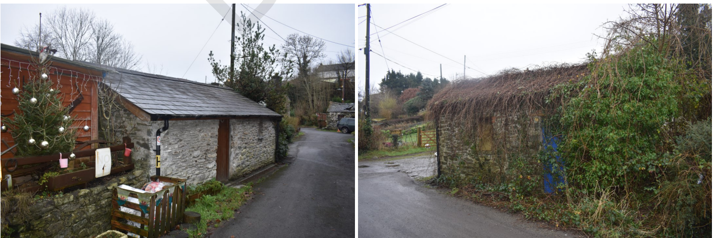
Figs. 24 and 25 Possible Ty Unnos with stone and slate replacing the original turf, cob and thatch
