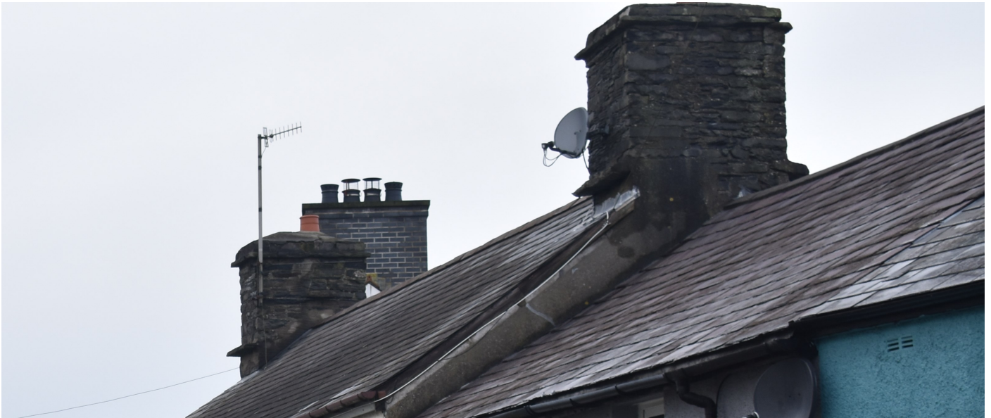
Fig. 22 Drip stones on some chimneys may indicate the earlier origins of some properties which might originally have had thatched roofs
