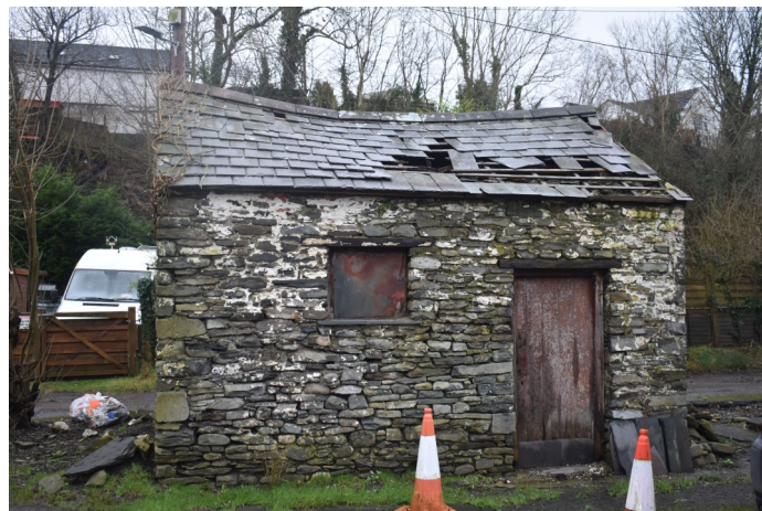
Fig. 19 Small vernacular stone barn (possible Ty Unnos?)
