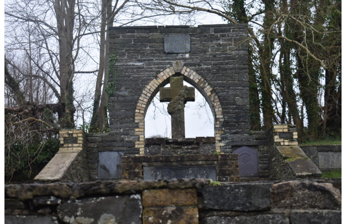
Fig. 15 Former Methodist Chapel
