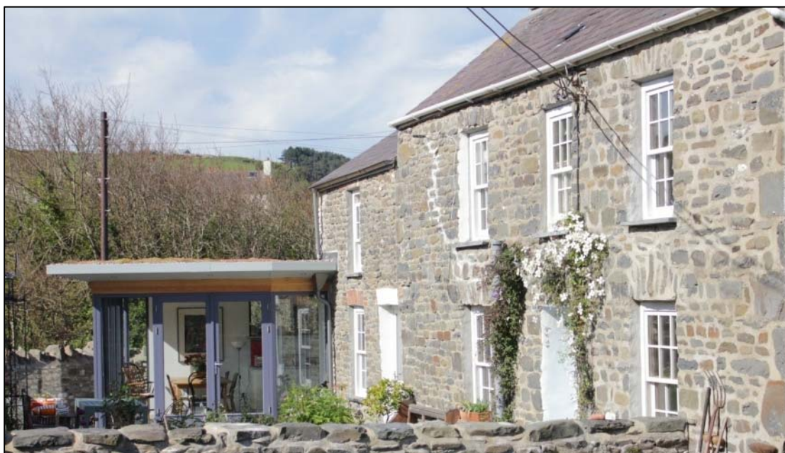
FIGURE 26: MODERN EXTENSION ON TRADITIONAL BUILDING Image: Courtesy of Zeta Freeman, Catalina Architecture.
