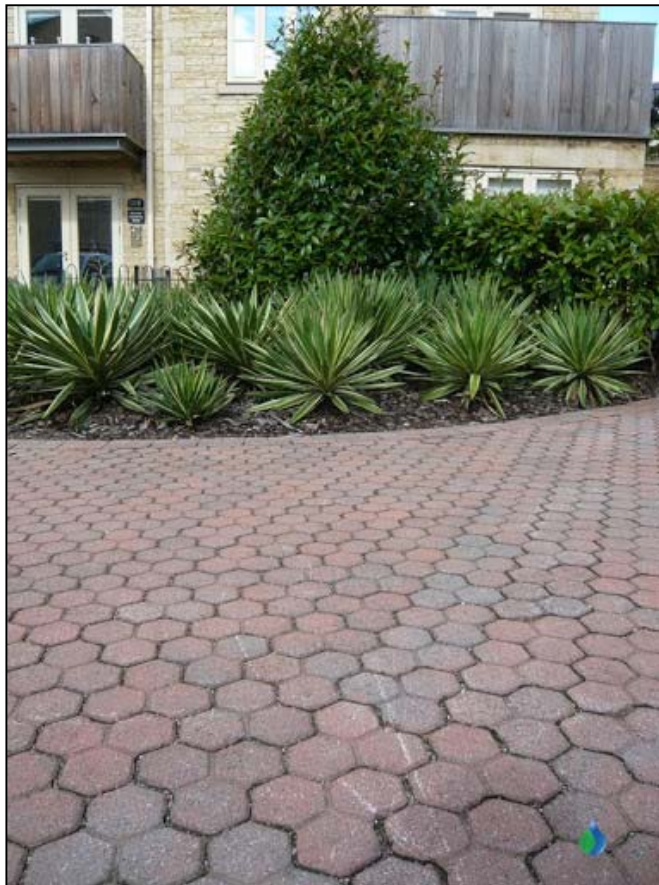
FIGURE 38: PERMEABLE PAVEMENT AT STAMFORD (SUSDRAIN)
