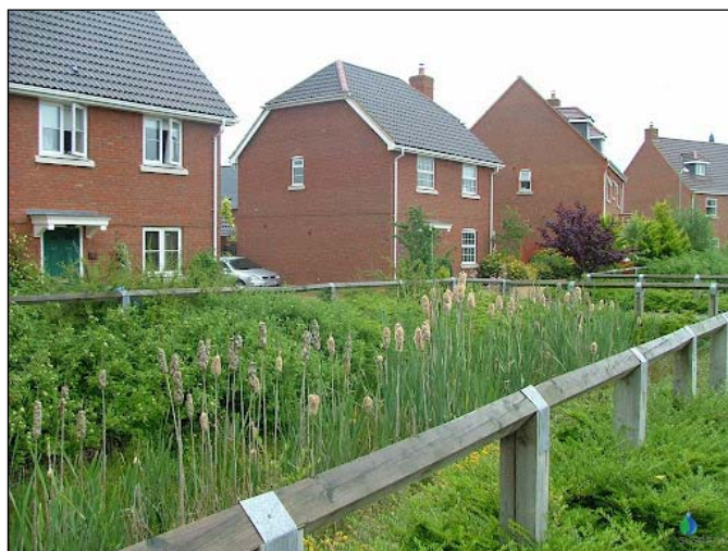
FIGURE 41: SuDS SCHEME ELVETHAM HEATH, HAMPSHIRE (SUSDRAIN)
