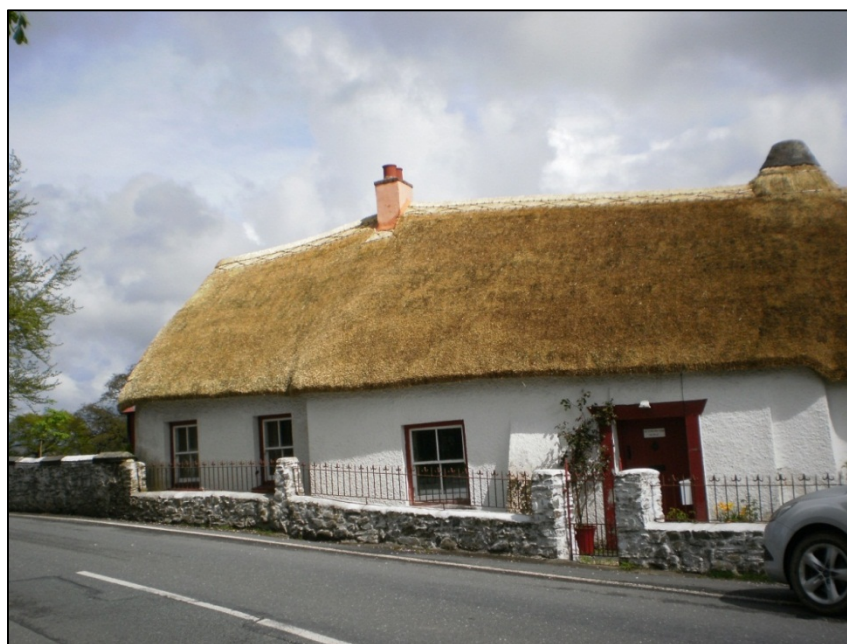
FIGURE 29: THATCH ROOF EXAMPLE WITHIN CEREDIGION
