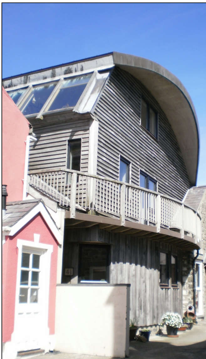
FIGURE 9: MODERN BUILDING WITHIN ABERAERON
