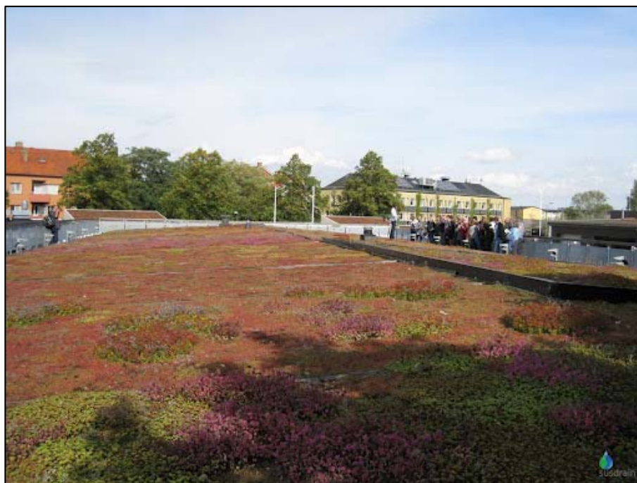
Figure 4: Augustenborg (Malmo) green roof center (Susdrain)
