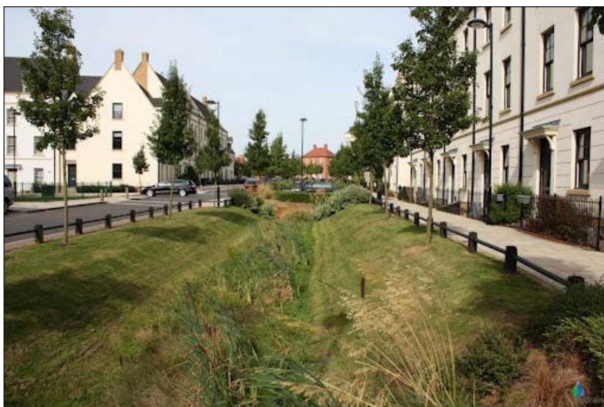
FIGURE 40: BLACK CAT DRIVE, UPTON, NORTHAMPTON (SUSDRAIN)
