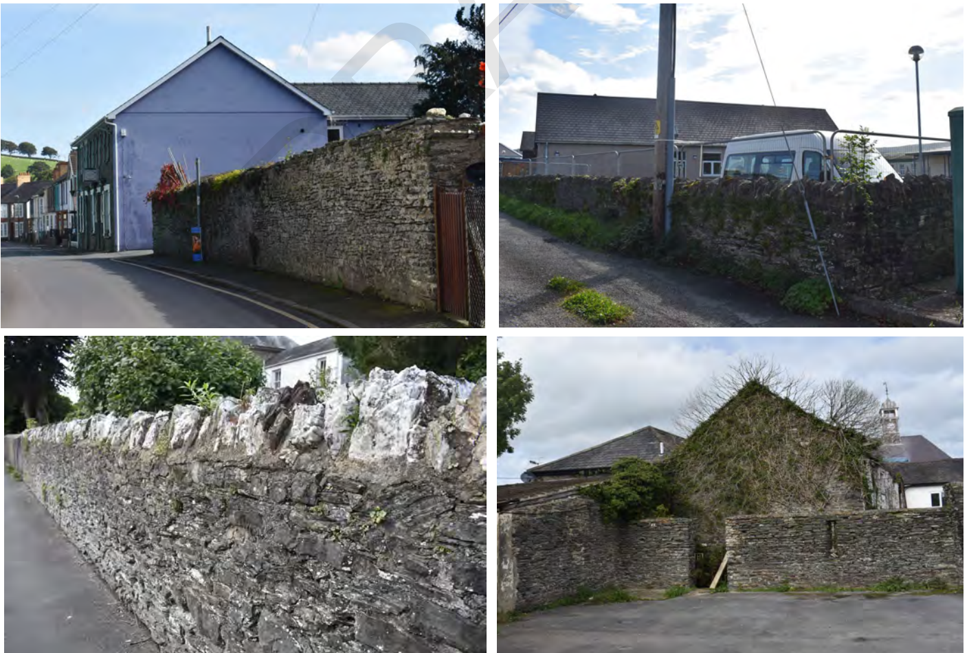
Figs. 14 to 17 examples of stone boundary walls within Lampeter town centre
