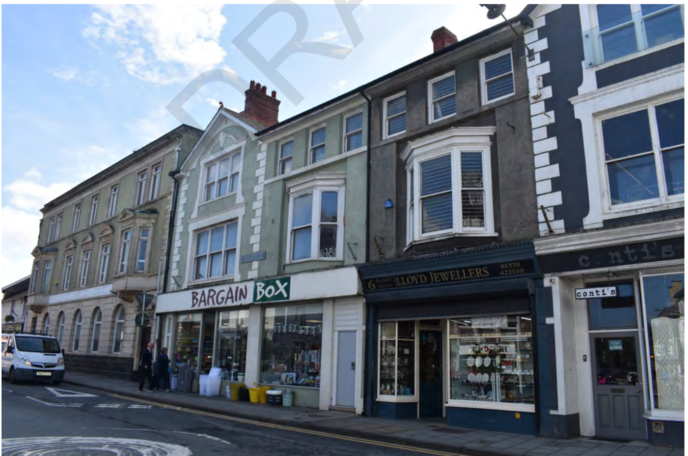
Fig. 46 The south side of Harford Square
