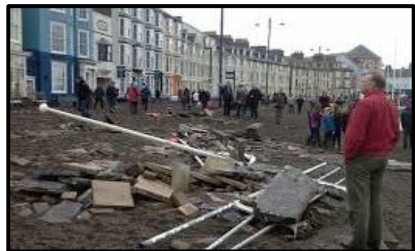
Cleaning the streets and repairing the roads
