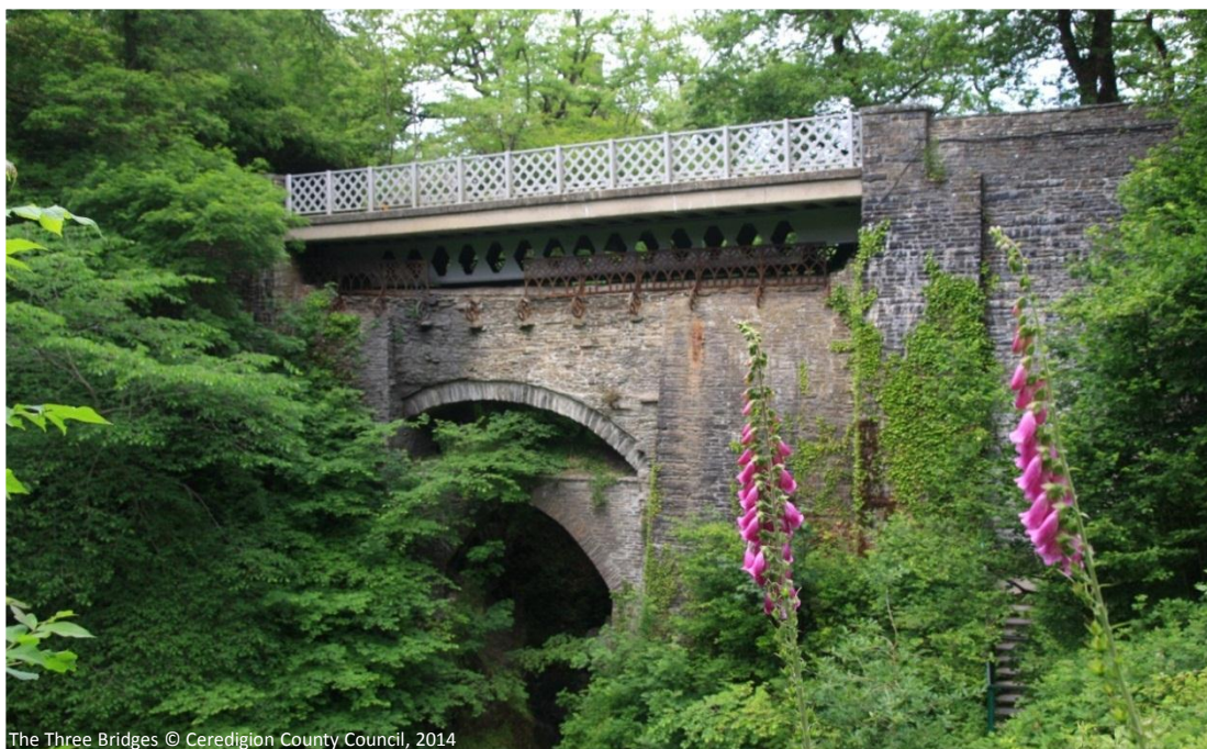
The Three Bridges © Ceredigion County Council, 2014
