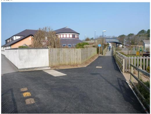
(AB14) Plascrug Avenue 'Phase 1' between Ysgol Gymraeg and Leisure Centre Shared use path widened to new Active Travel Design Guidance standards. 2 number raised table crossings installed. Steel bollards installed to provide safety for cyclists and pedestrians and prevent vehicle parking on paths.
