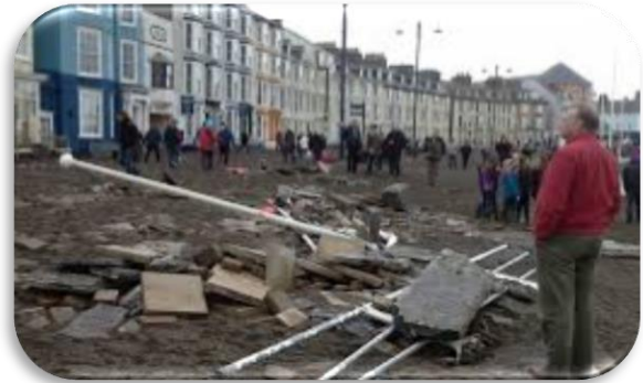
Cleaning the streets and repairing the roads
