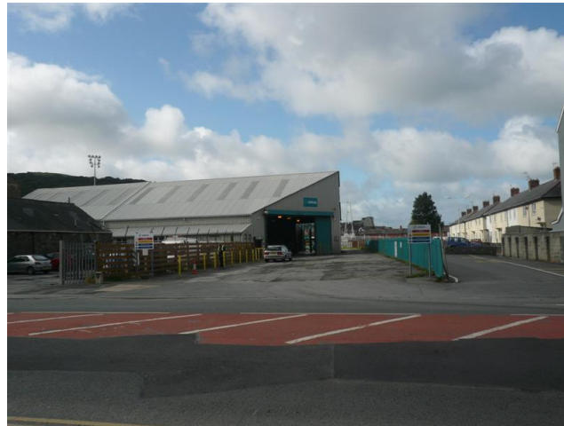
Fig 14 Arriva Bus Depot, Park Avenue South
