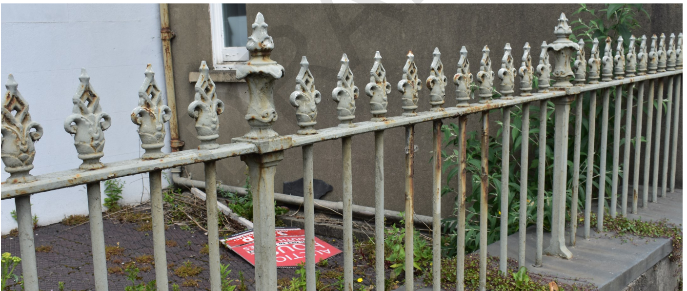
Fig. 24 Original cast iron railings
