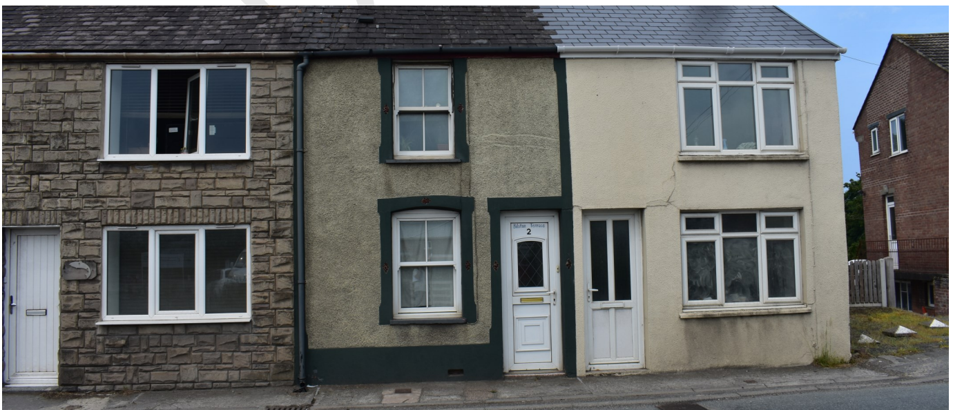
Fig. 2 The loss of traditional windows and doors, cladding and cement render negatively affects the character and appearance of traditional cottages
