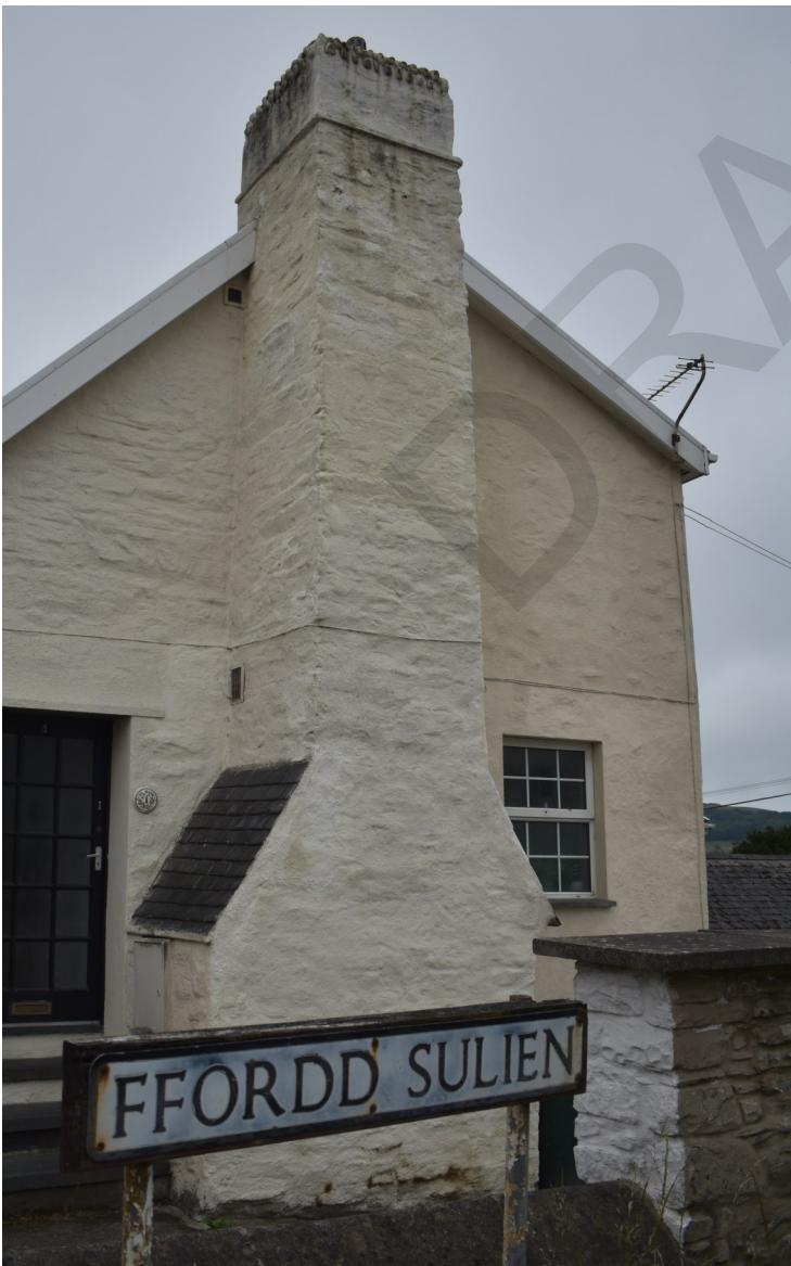
Figs. 21 and 22. The chimney dimensions on Tymawr (left) and Tan Y Fron (below) indicate their earlier origins
