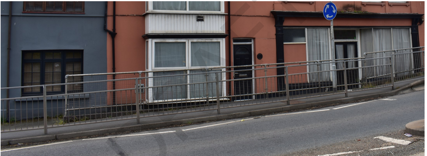
Fig. 28 Inappropriate utilitarian safety railings
