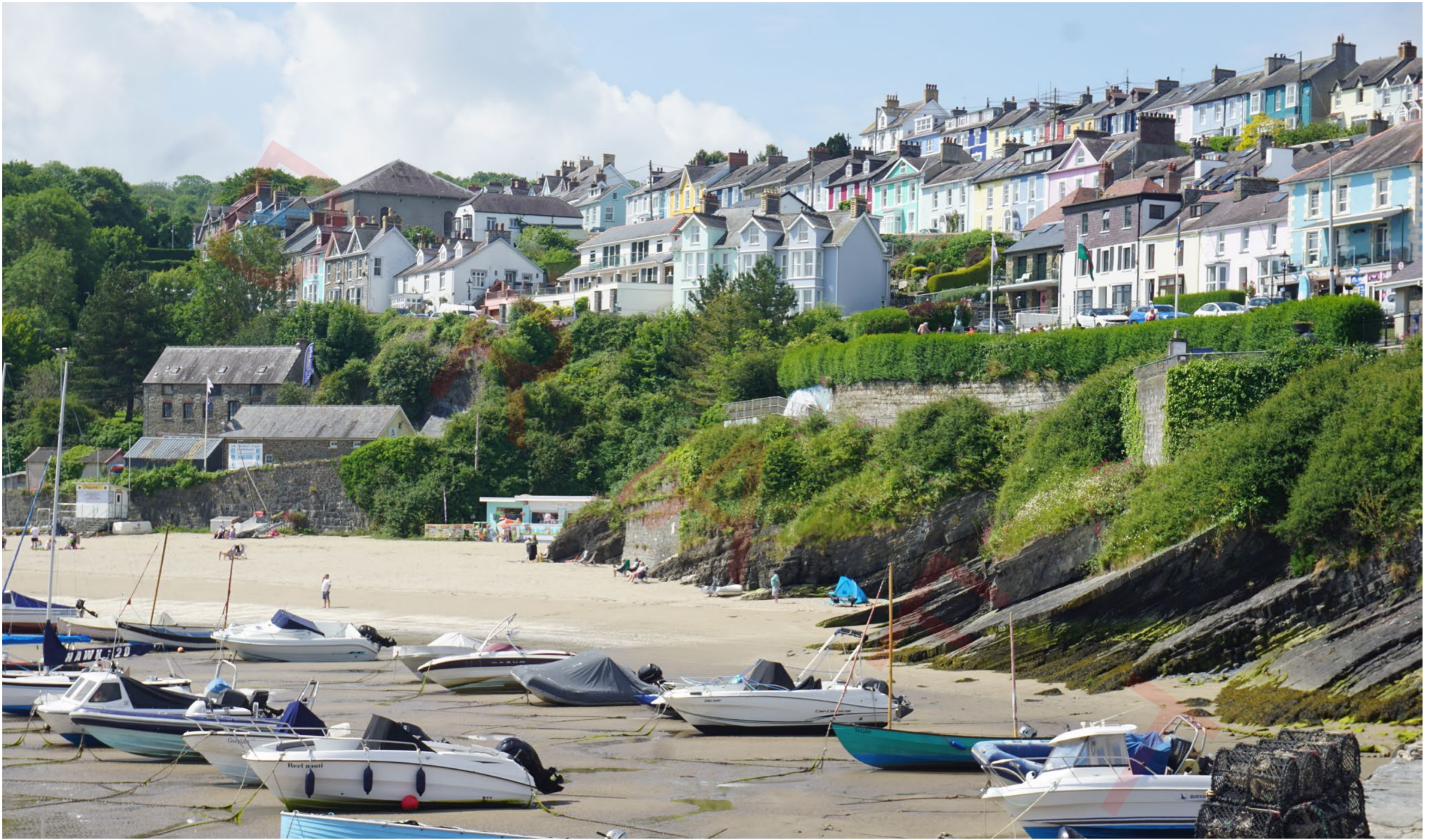
New Quay Harbour
