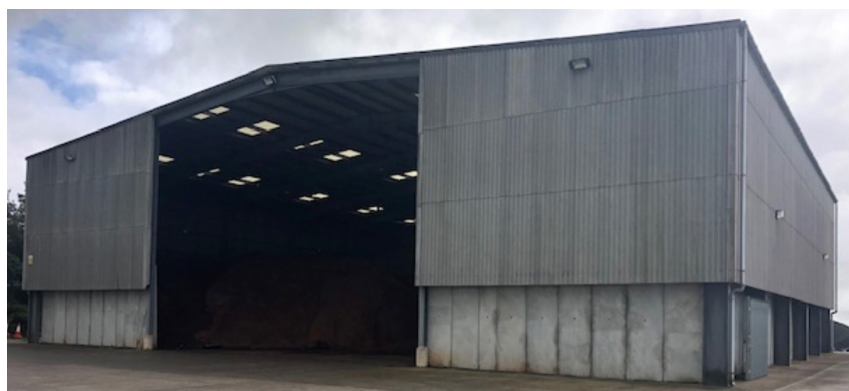
Figure 18 – Salt Barn at Penrhos Depot, Llandysul. Capacity = 6,400 tonnes
