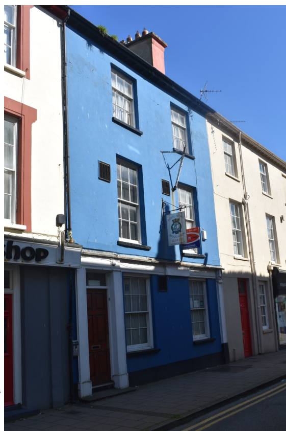
Fig. 11 Georgian town houses in Market Street
