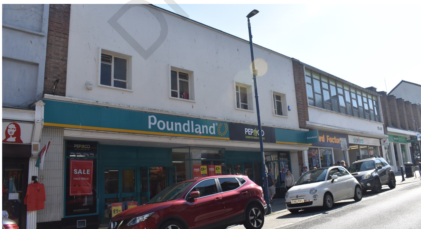
Fig 13 Poor quality 20th century redevelopment in the town centre
