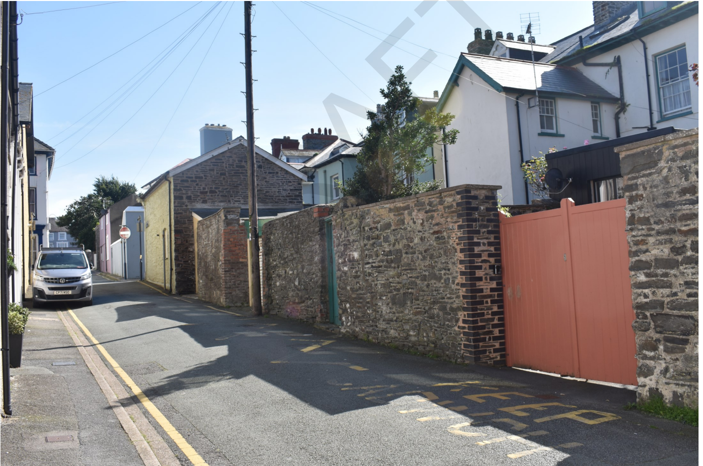
Fig. 32 Rear yard areas, especially in the old town, may reveal evidence of former land use
